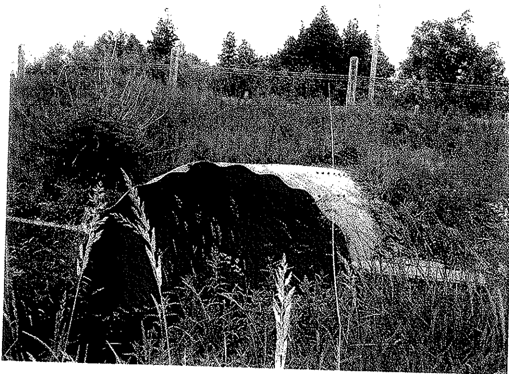
Culvert requires some backfill to support new trail
